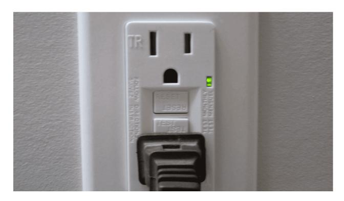
GFCI stands for <u>Ground Fault Circuit Interrupters</u>. In simple terms, this is just fancy electrical protection that prevents you from being shocked. That's why **NEC** (National Electrical Code) requires GFCI protection for every room at a home that is close to a water source.
